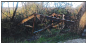
May: Rusty Old Railroad Bridge Stirs Intrigue in Majors Park
