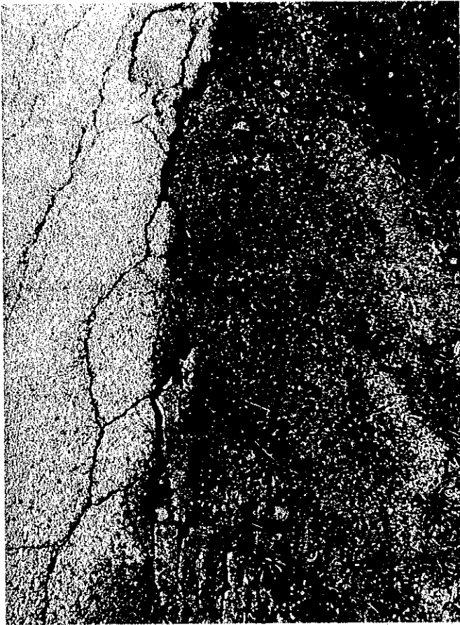
Edge Cracking on Boies Rd.
