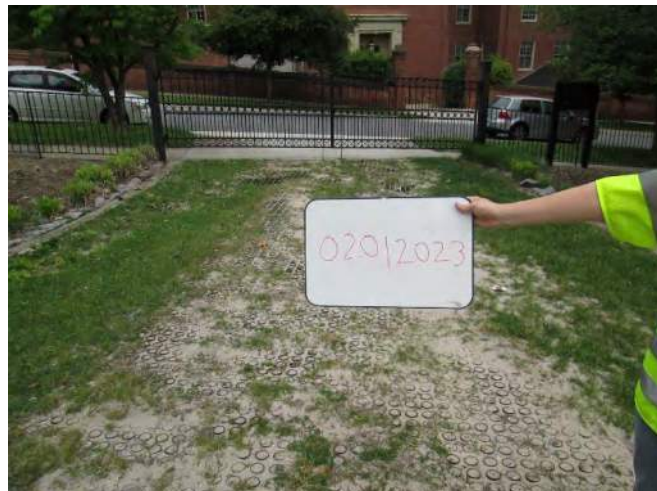
Figure 3.2. A white board and digital camera can be handy to note SMP tracking #, date of inspection, and other forms of documentation. Note that an inspector may alternatively tag photographs, particularly if they are recorded on a smartphone or Tablet.
