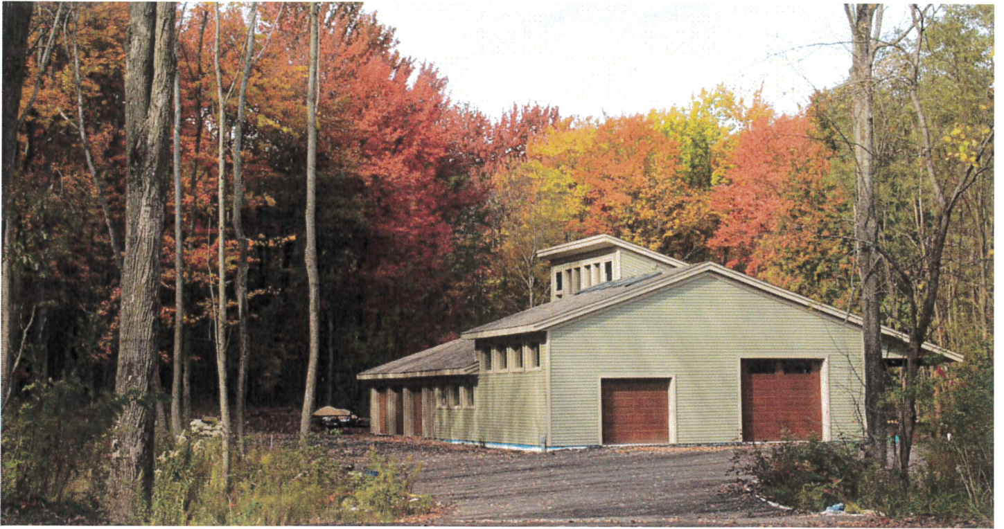
View of Dwelling from Midpoint of Existing Driveway – Fall 2018
